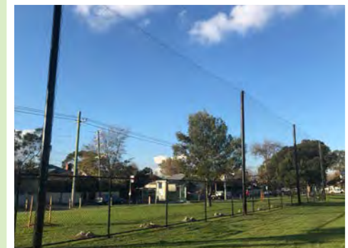
Existing high ball stop fence
