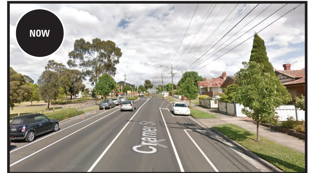
Existing conditions: 2-way vehicle movement, dedicated bike lane (no buffer) marked parallel parking, grassed nature strips and footpaths to both sides of the street.
