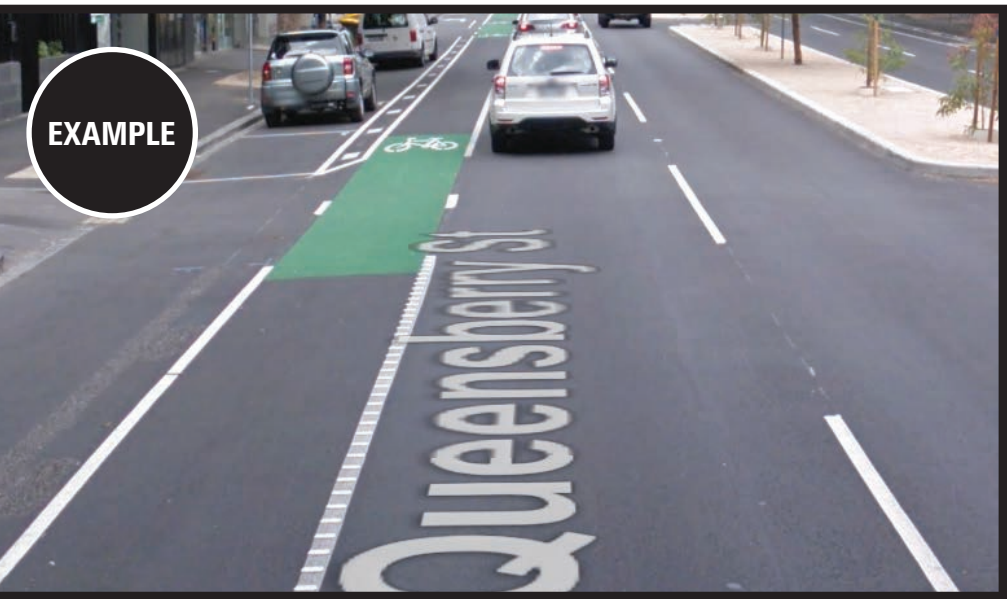
Example of dedicated cycle lane with buffer & tactile pavement marking to raise driver awareness along Queensberry Street, Melbourne.
