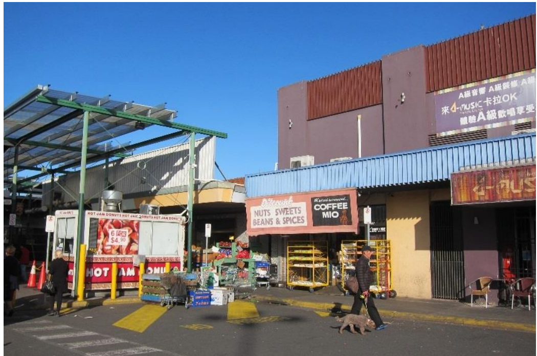
Figure 24. View of the eastern edge of Shed 2. On the left of the image, single storey brick buildings have shop fronts facing the pedestrian walkways and a propped tall metal parapet. On the right of the image, double storey masonry buildings have shops at ground level and solid masonry walls to the upper storey. (Source: Context 2017).
