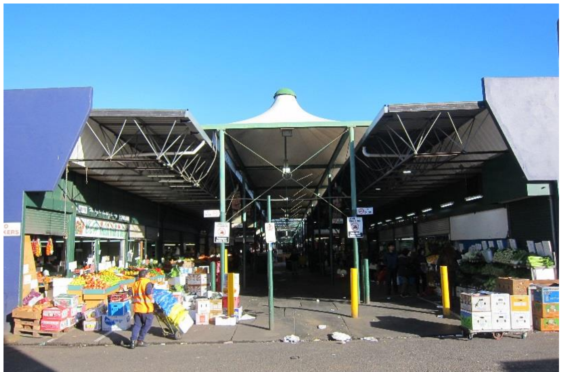
Figure 33. View from the eastern edge of The Centreway showing the canopy structure inserted between the open space and the shed roofs. Original space frames are visible. The prefabricated concrete panel end walls reflect the outline of the space frames. (Source: Context 2017).
