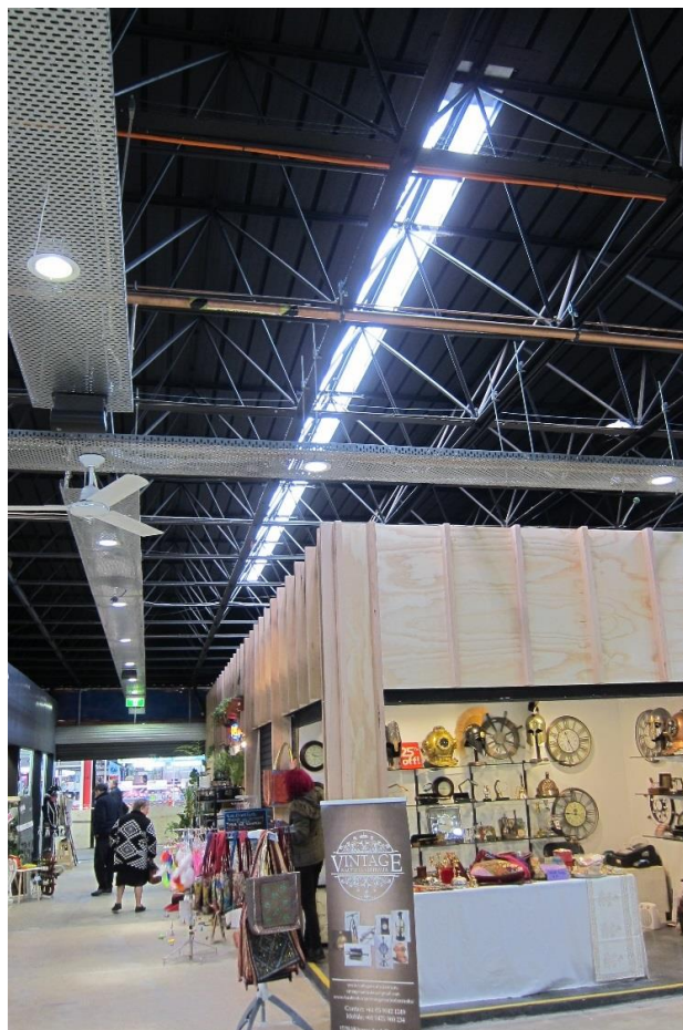
Figure 21. Internal view of Shed 1 showing recent updates including painted space frames and flexible wall partitions. (Source: Context 2017).
