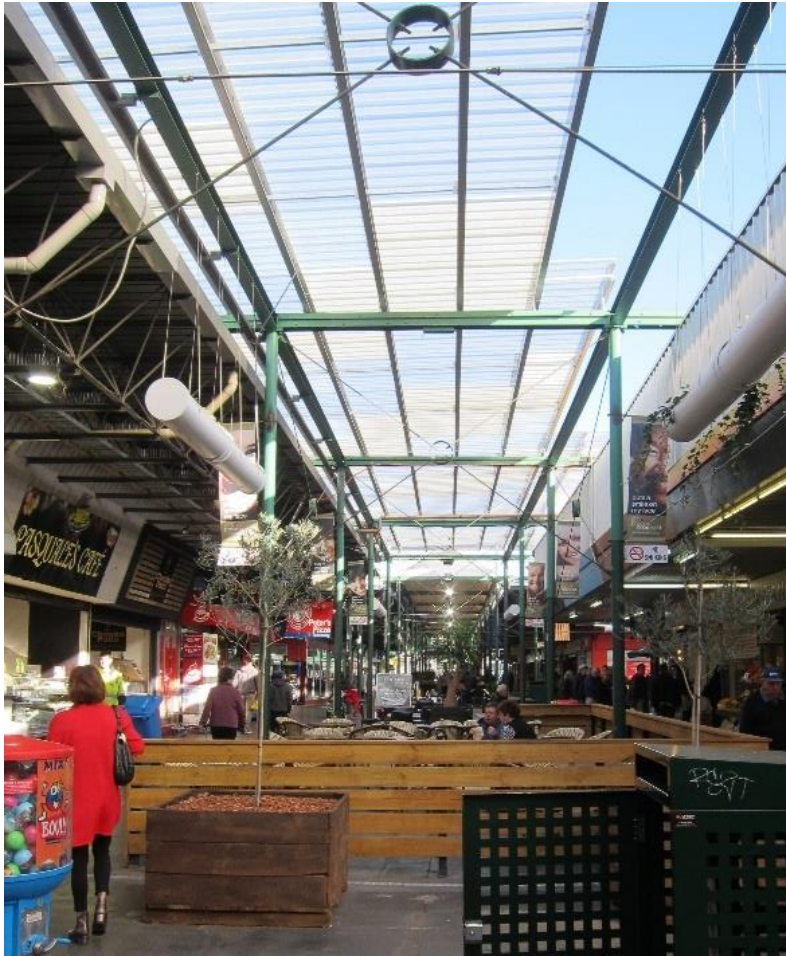
Figure 34. Opaque pyramidal canopies have been replaced with clear corrugated material in certain sections of the Market (Source: Context 2017).
